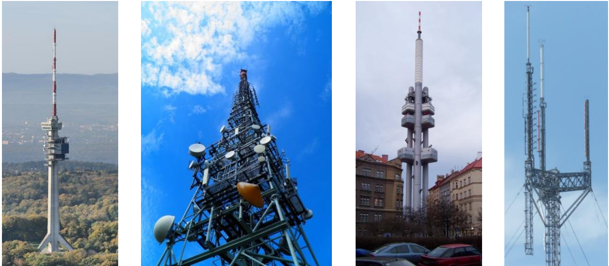
Figure 1: Typical broadcast towers
