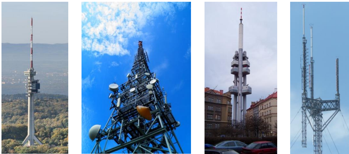
Figure 1: Typical broadcast towers (Europe and USA)
